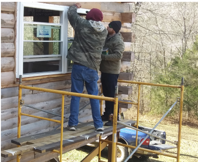
Windows being installed in dinning hall
